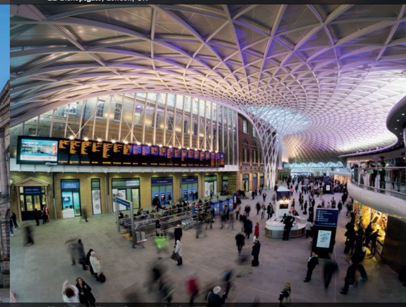
King's Cross Western Concourse, London, UK
