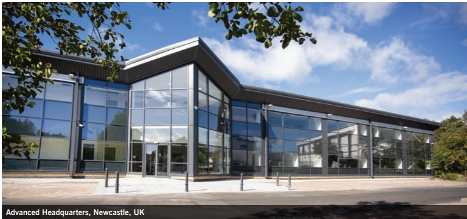
Advanced Headquarters, Newcastle, UK
